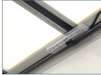
Light strip roof made of aluminium cross slats covered with light transmissive GRP panels
